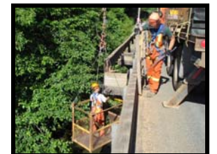
Dwayne Randall in basket and Mitch Jensen installing safety rails.
